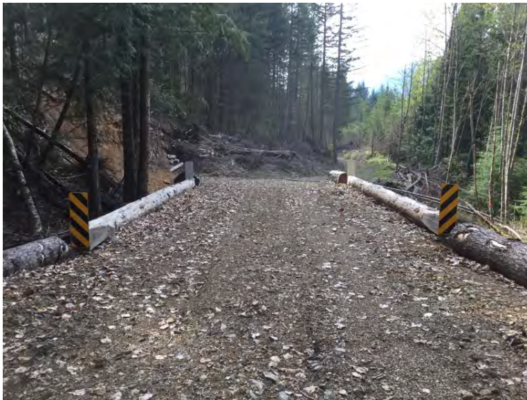
Approach from Right Bank when facing downstream
