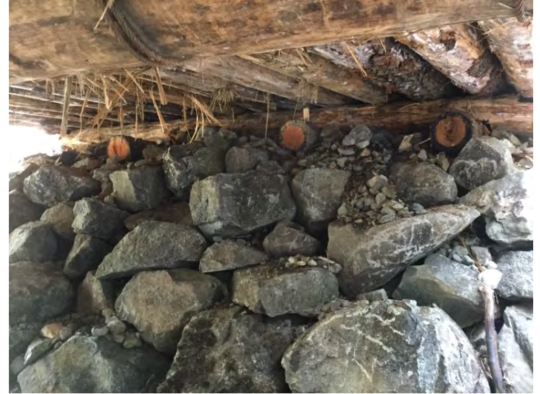
Right Bank Abutment when facing downstream
