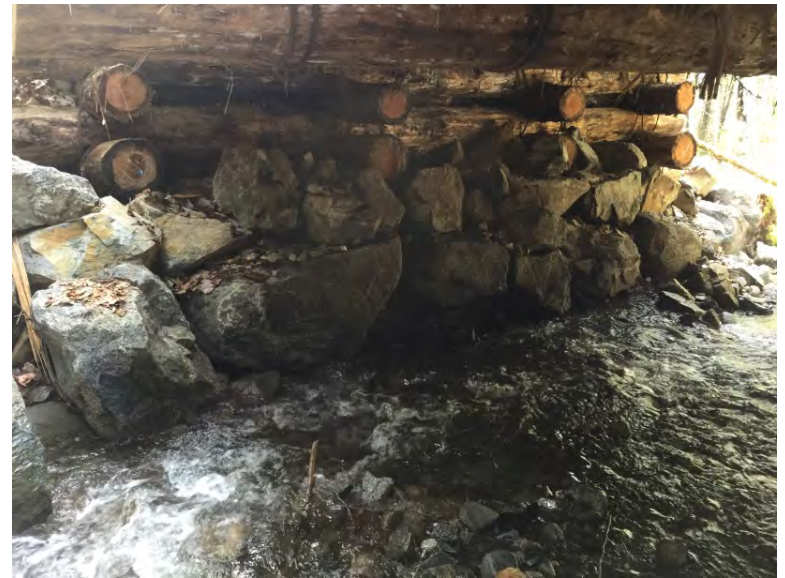
Left Bank Abutment when facing downstream
